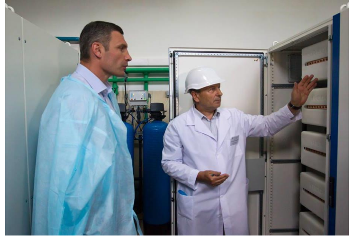
Waterwork Ukraine with REDO Installation
