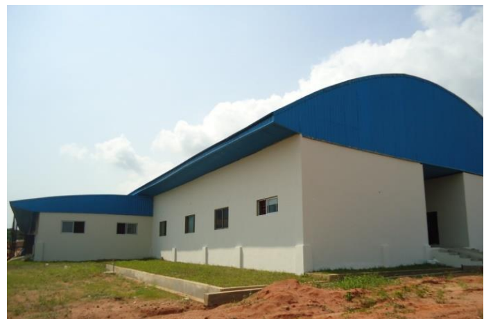
Waterwork Nigeria with REDO Installation
