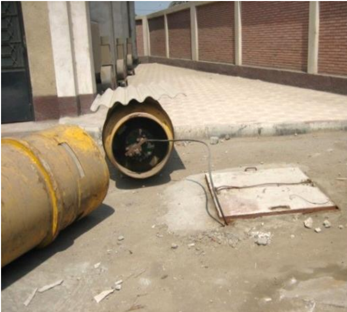
Before: disinfection with chlorine gas
