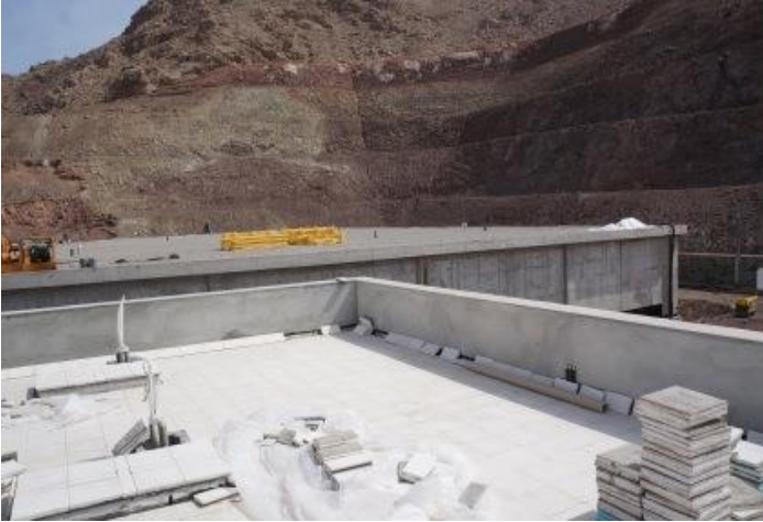
Waterwork Oman with REDO Installation
