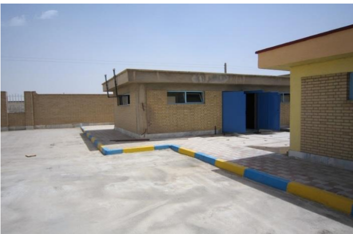
Waterwork Iran with REDO Installation
