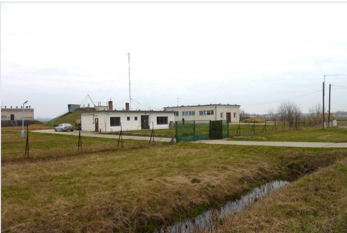
Waterwork Hungary with REDO Installation
