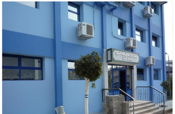
Waterwork Egypt with REDO Installation
