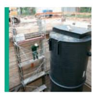
**The material in the durable sump pumps is: PE-HD** We place emphasis on proven durability to safeguard your requirements on a sustainable basis – with thermoplastic PE HD (high density polyethylene).
