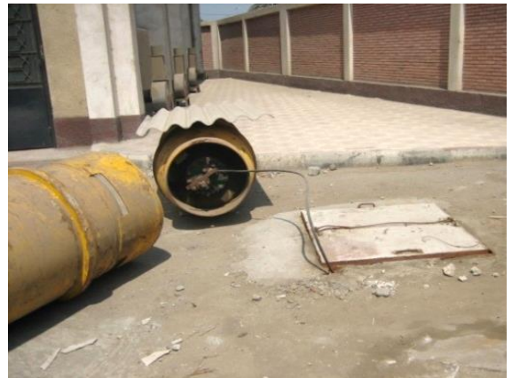
Before: disinfection with chlorine gas
