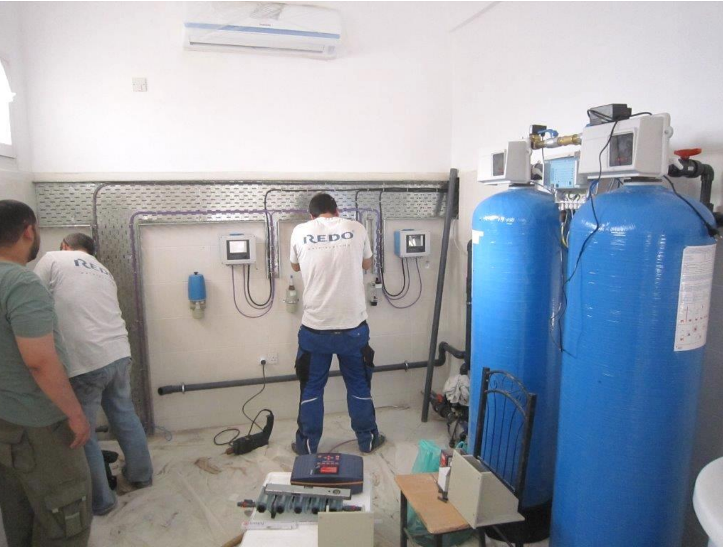
REDO Installation Waterwork
